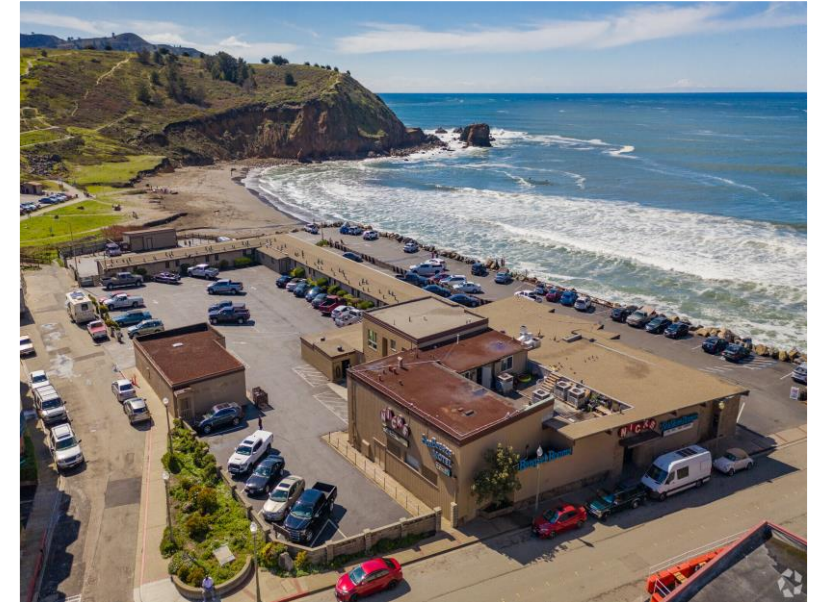
Nick’s restaurant beach erosion
