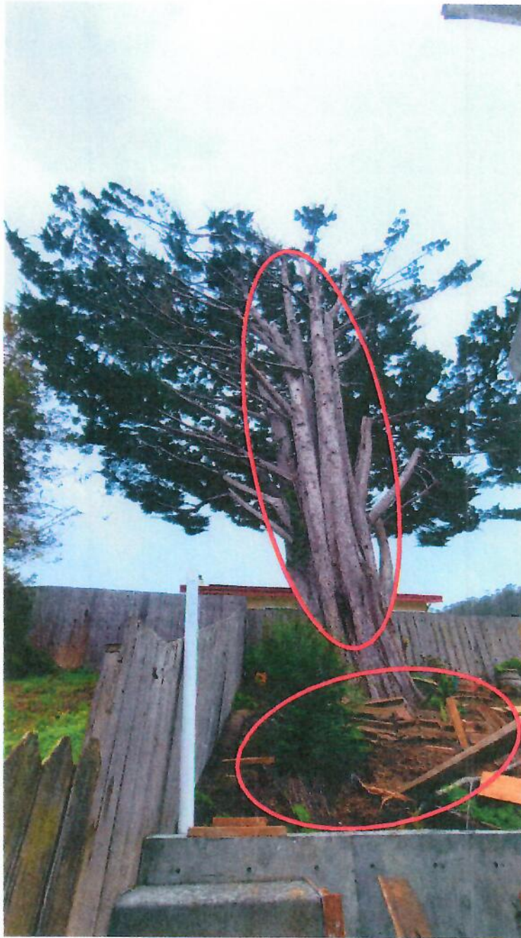
Leaning one-sided tree with multiple co-dominant stems – prone to failure Compromised structural root zone
