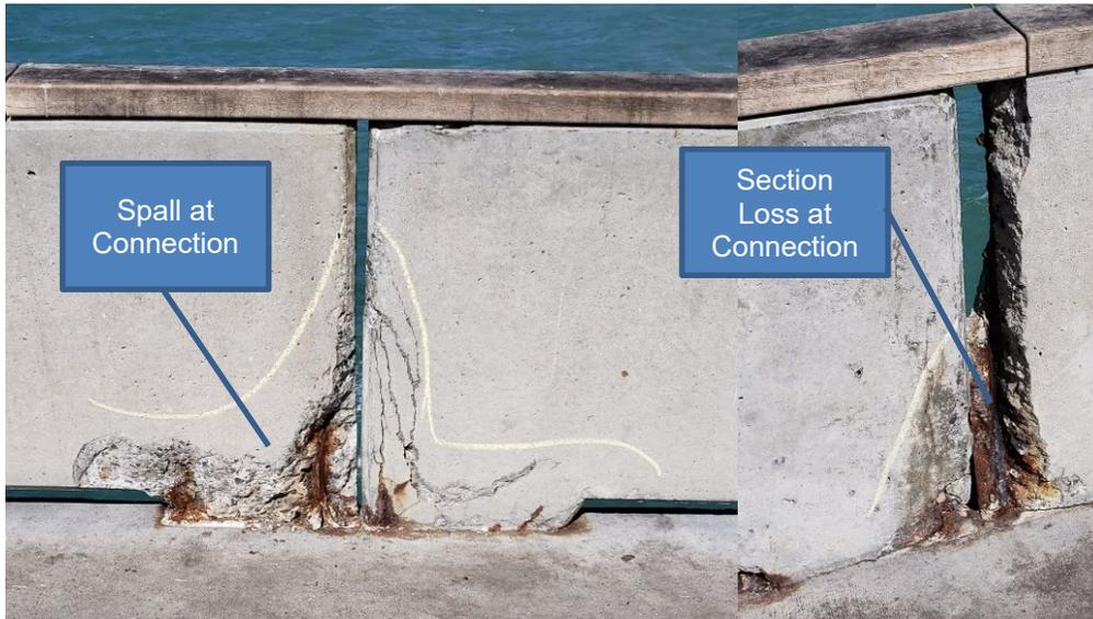
**Figure 8: Typical Damage Rated Severe**
