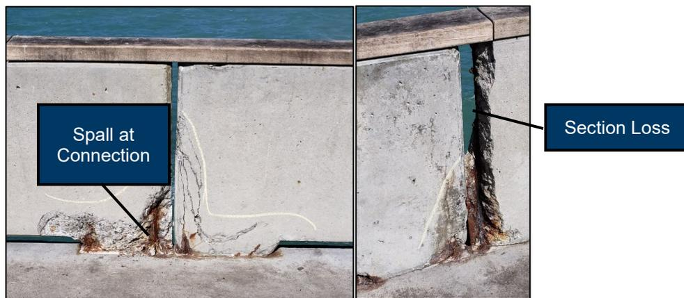
Figure 3.5: Typical Damage Rated Severe
