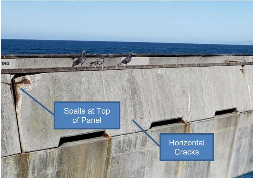
**Figure 6: Typical Damage Rated Moderate**
