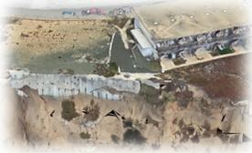
RJR has been working in this area of Pacifica, California since the late 1990's with specific work on this bluff since 2008 to the present. We understand the City is proceeding with a seawall design that will connect to the existing sea wall north (Ocanaire)<sup>1</sup> and south to the sea wall at 360 Esplanade Avenue (Almco). In principle, in the opinion of RJR this is a prudent approach to retard bluff retreat. However, RJR has the following comments.
