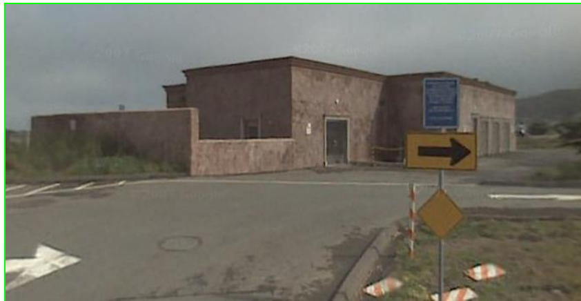
Linda Mar Pump Station (Drainage)
