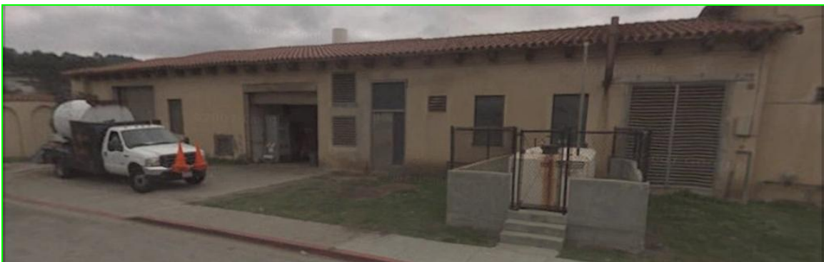
Sharp Park Pump Station
