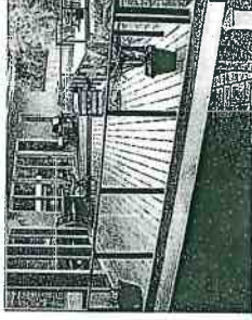
Grand Rail Fence: Black anodized aluminum with structural glass panels, 42" high
