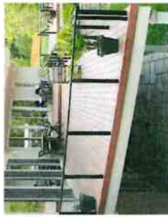
Ground Rail Detail: Black anodized aluminum with structural glass panels, 42" high
