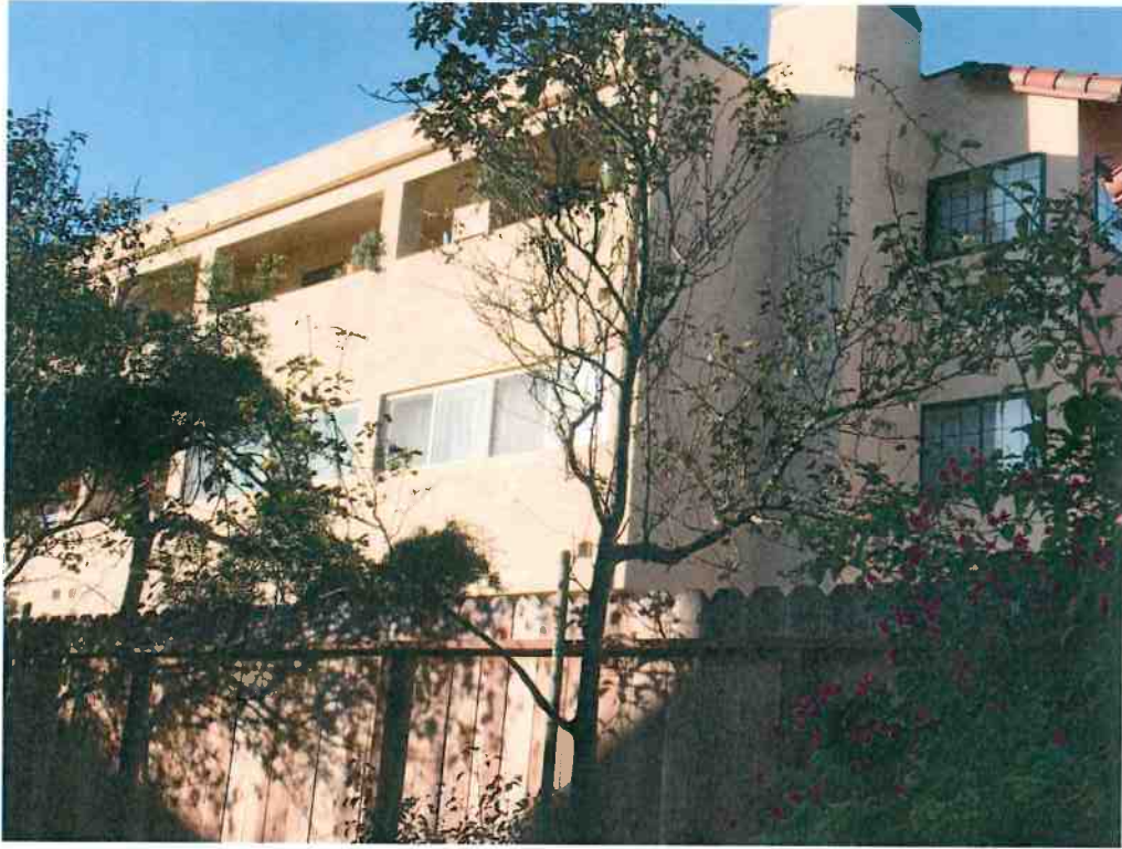
Figure 3. Closer view of Development
