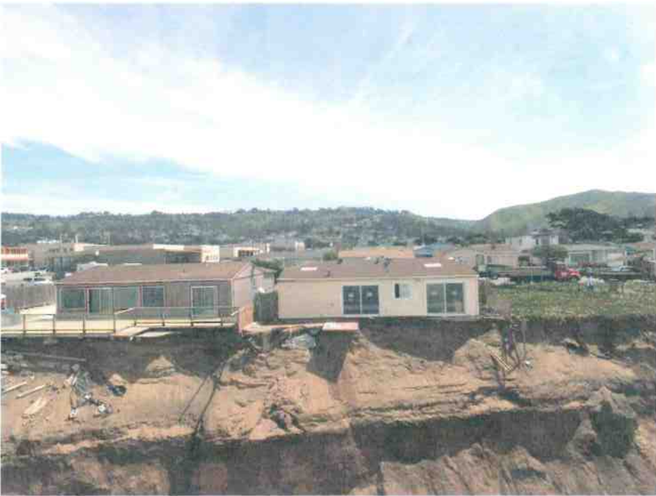
Level view of back of 532 Esplanade Avenue pre house move
