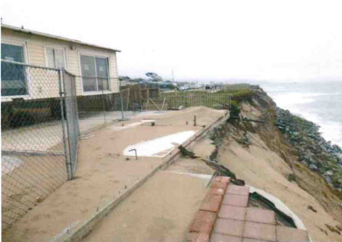
Rear view of 532 Esplanade Avenue, post house move
