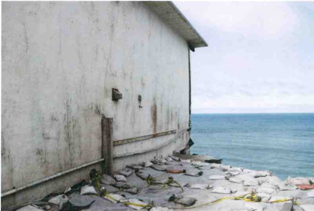
Photo 3A – North Side of 330 Esplanade Building
