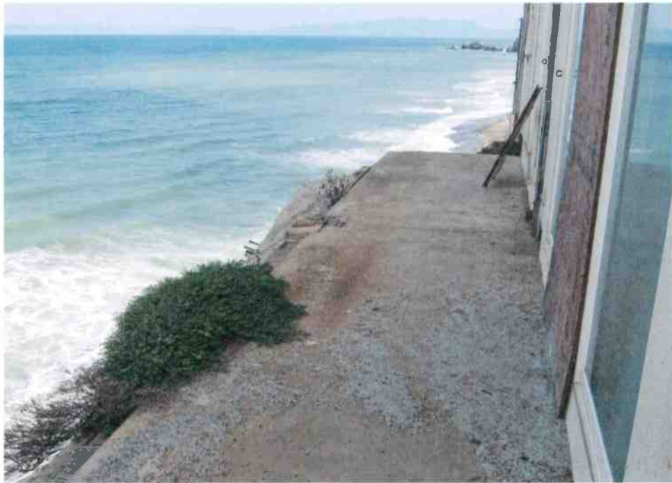
Photo 1B – 330 Esplanade Northern Patio
