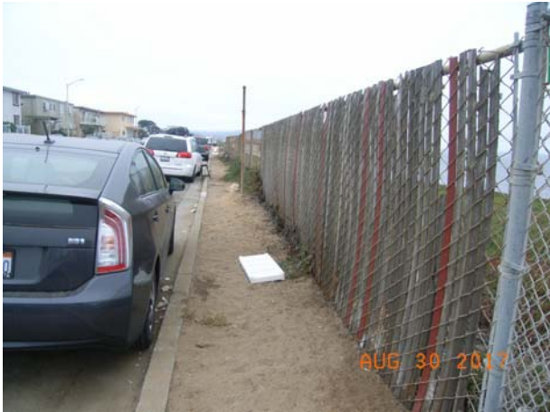
Figure 6D. Existing seaward edge of Esplanade Avenue, showing existing chain link fencing, looking southerly.
