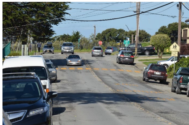
The existing mid-block crossing on Monterey Road near Ocean Shore School.
