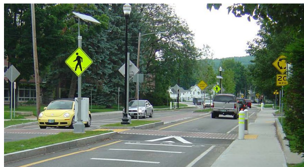
An example of a raised crosswalk.
