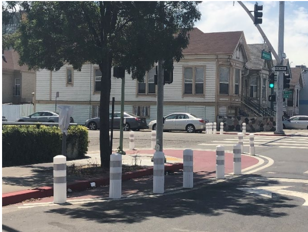
A paint-and-post curb extension in Oakland.
