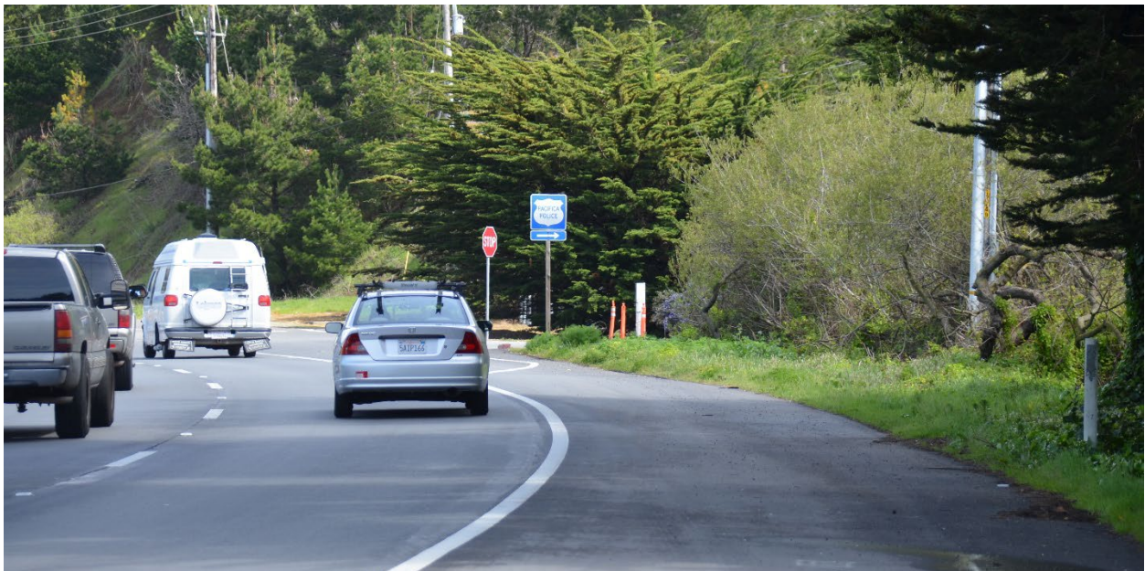
Highway 1 south of the Pacifica Police Station, highlighting the lack of non-vehicular access to the station.
