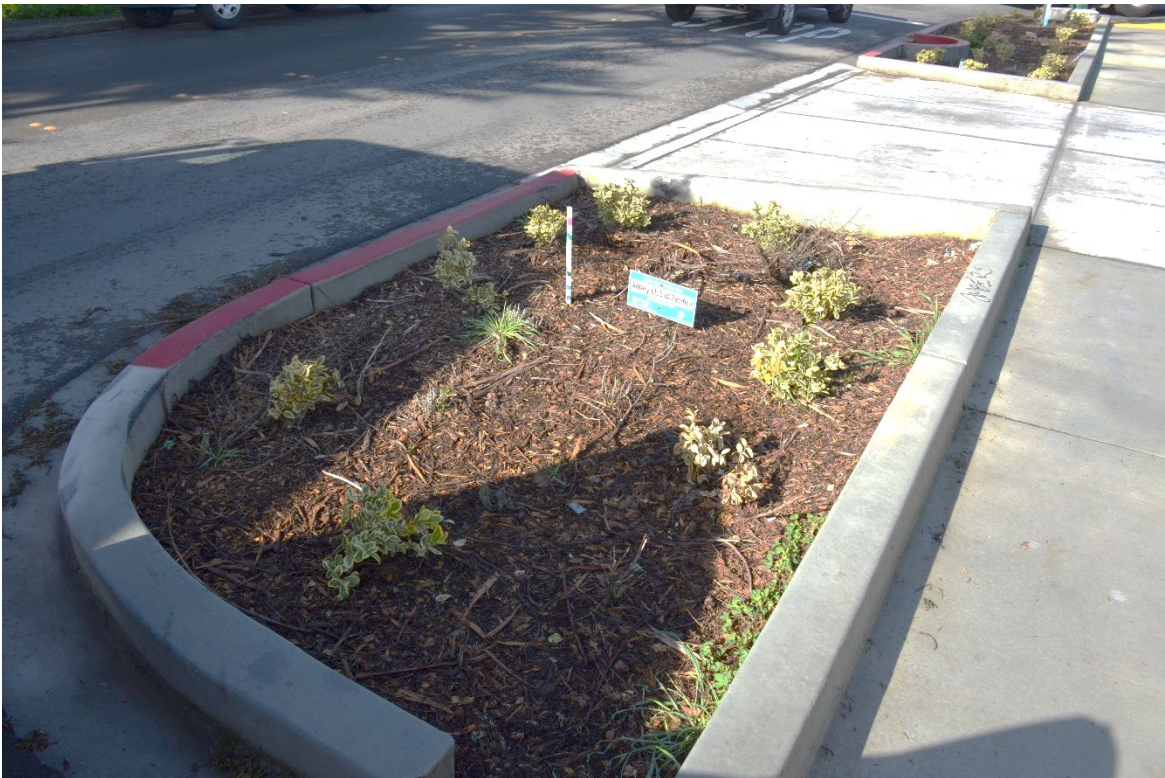
Newly installed green infrastructure along Palmetto Boulevard.
