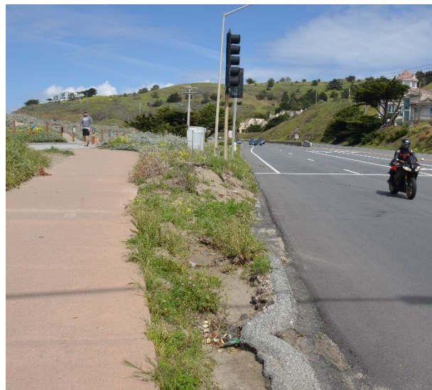
The separation between the Coastal Trail and Highway 1 at the Crespi Drive intersection.
