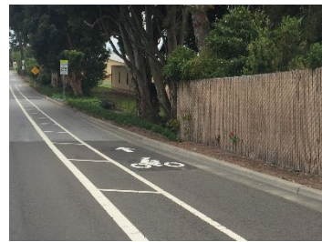
Class IIB Buffered Bicycle Lane
