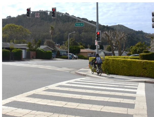
The southern crossing of Peralta Road at Linda Mar Boulevard with a student biking on the sidewalk. The high bushes significantly affect visibility around corners.
