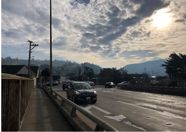
The Manor Drive overcrossing.
