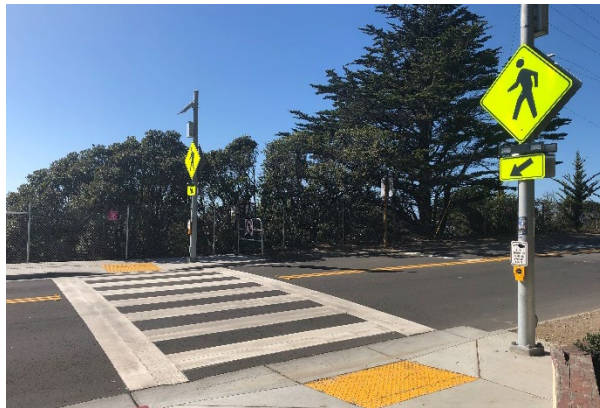
An RRFB at a mid-block crossing across Oceana Boulevard.
