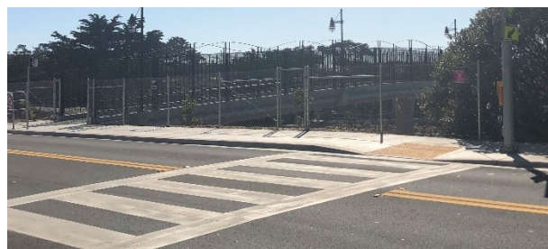
The recently constructed pedestrian overpass near the Eureka Square Shopping Center.
