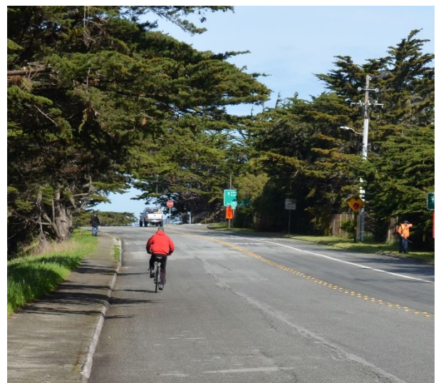
Underutilized roadway space can be used to construct bicycle facilities to facilitate safe, more comfortable travel.
