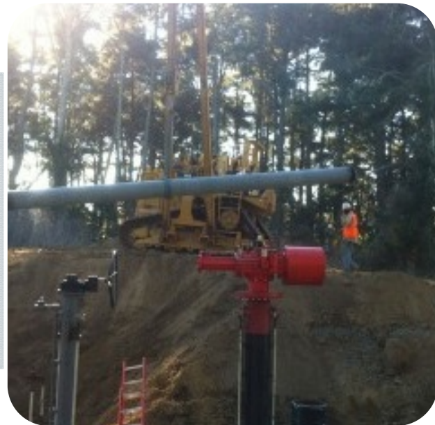
Infrastructure Upgrades Valve Automation
