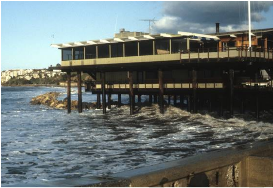
Santa Barbara Yacht Club, beach and parking lots flooded during 1983 El Niño, elevated sea level and storm waves. (Photo credit: Gary Griggs)
