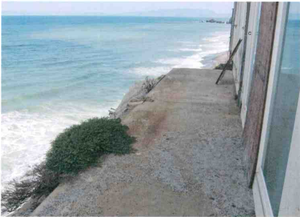
Photo 1B – 330 Esplanade Northern Patio
