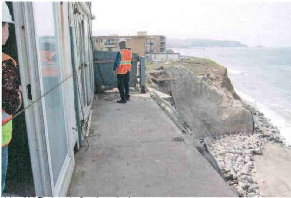
Photo 1A – 330 Esplanade Southern Patio
