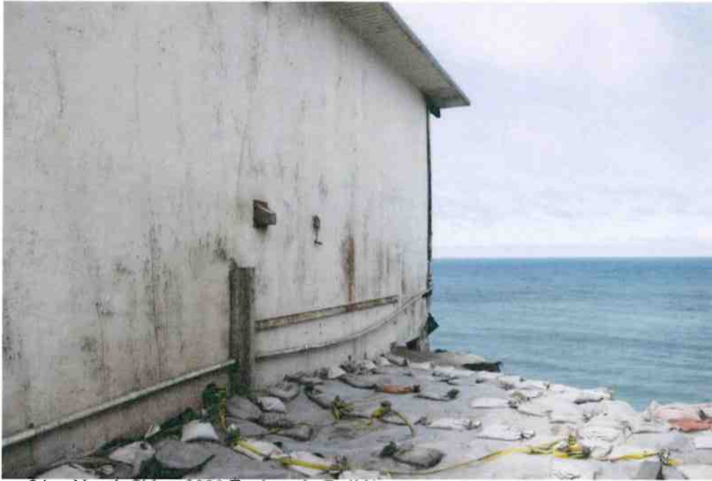
Photo 3A – North Side of 330 Esplanade Building
